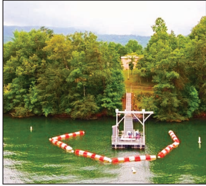
The Hiwassee Water Treatment Facility pulls water out of Lake Chatuge to treat for drinking and other uses. Photo/HiwasseeGA.gov
